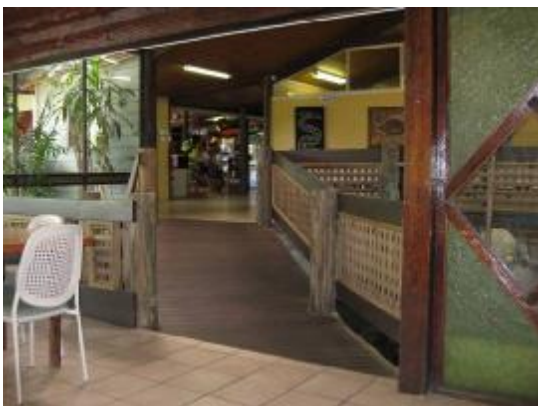
Small Ramp leading to Reception area
