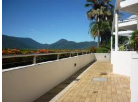
View over Trinity Inlet from path leading to ramp
